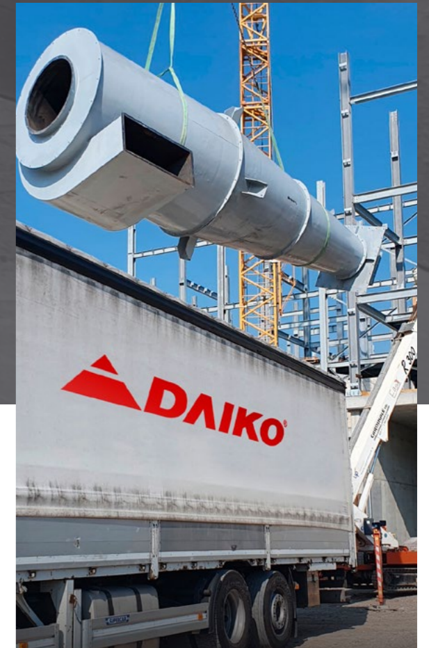
Cyclone delivery at construction site
